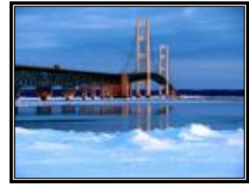
Mackinac Bridge (picture from www.mackinacbridge.org/photo-gallery )
